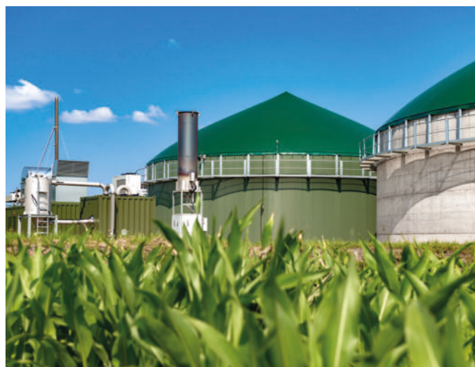
Agricultural biogas plant
